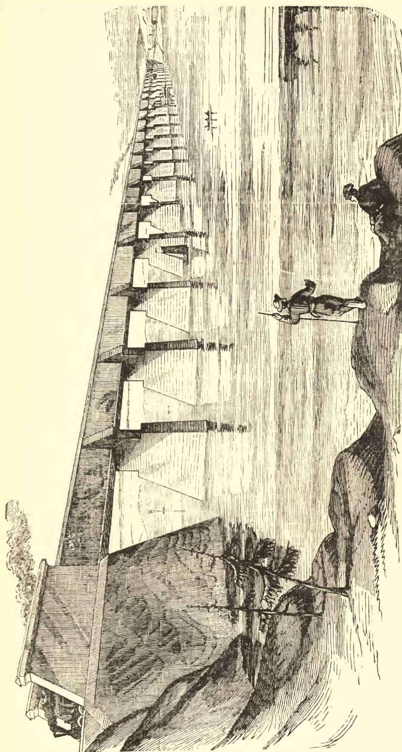
THE VICTORIA TUBULAR BRIDGE, ACROSS THE ST. LAWRENCE, MONTREAL. TOTAL LENGTH WILL BE 10,284 FEET, OR ABOUT 50 YARDS LESS THAN 2 MILES—NOW BUILDING.
